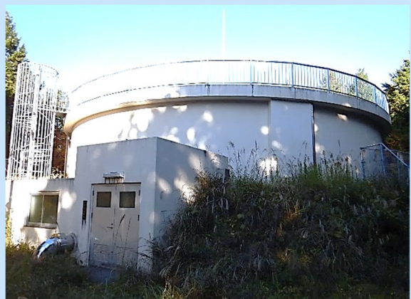
伊里前配水池 (1,000m 3 )
